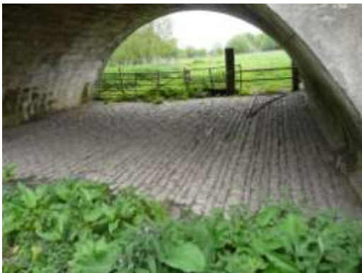
Paved arch under the bridge
