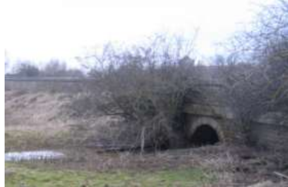
The culvert - north end of the drain
