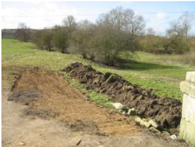
Work started on footpath slope
